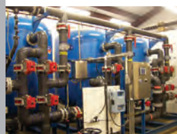
biotta biological filtration system from AdEdge Water Technologies
