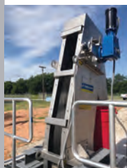
SAVI GVS Multirake Perforated Plate Screen from Enviro-Care
