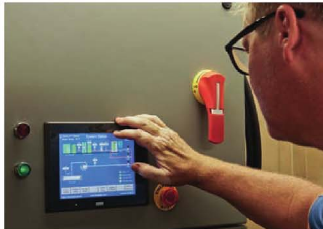
Left: Wastewater technician monitors and controls FORSe and Phantom systems using remote digital telemetry. Photo by Anue
