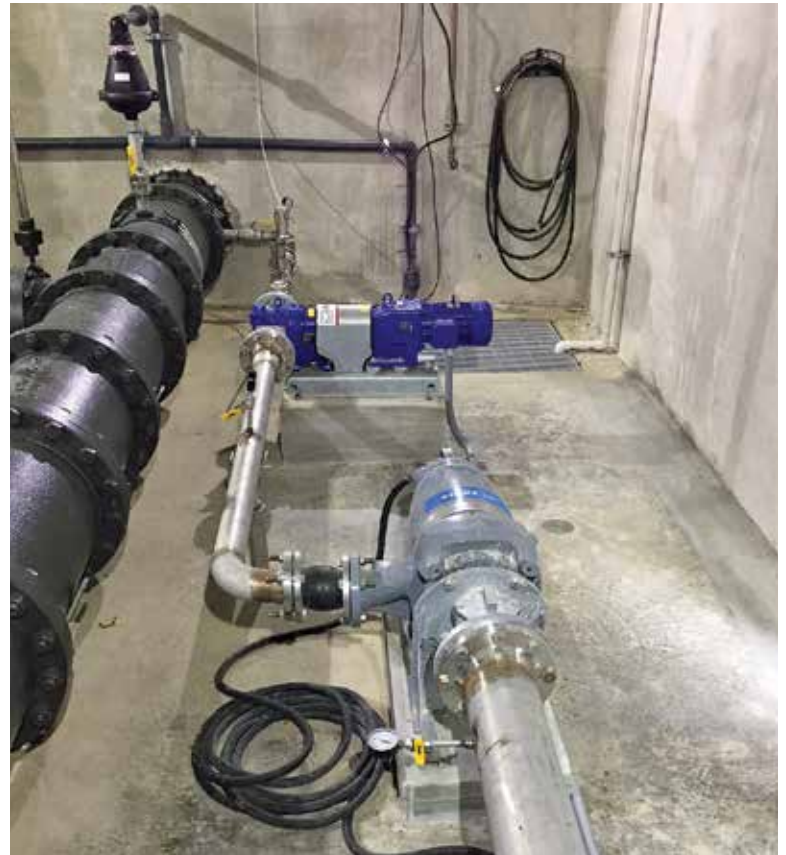
The system’s main components include a high-volume air compressor, an oxygen concentrator that takes in ambient air and produces a dry and purified stream of oxygen, and an ozone generator that receives the purified oxygen and produces ozone at an average concentration of 5 percent by weight.
