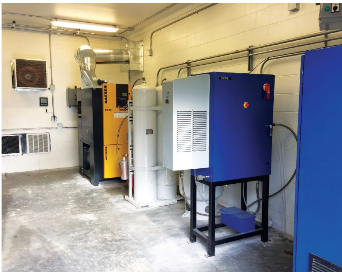
Oxygen and ozone odor control systems inject the elements into the treatment train to kill sulfide, reducing bacteria that create the characteristic odor associated with wastewater treatment plants.
