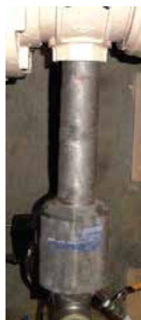
Picture 2: Tapped Force Main with Attached Infuser
